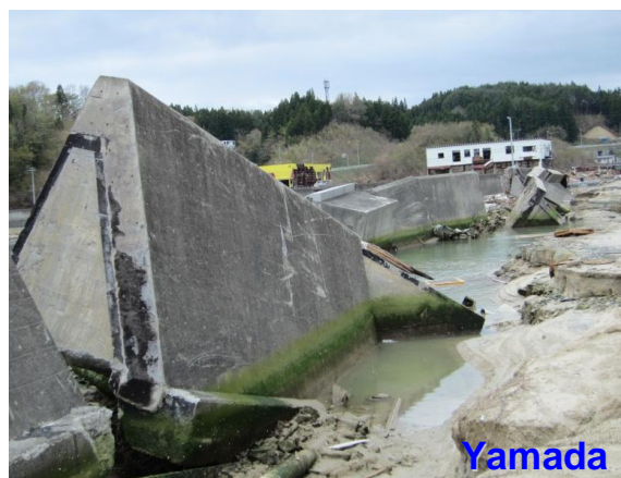
Destruction by tsunami scouring
